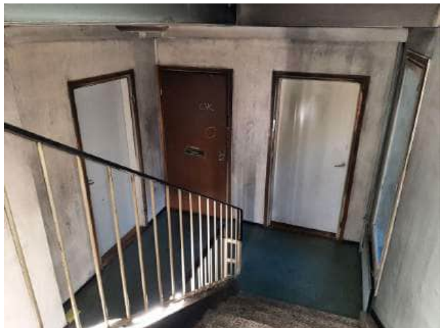
2krs, as 10 ja as 12 rikutut ovet irrotettu kokonaan
