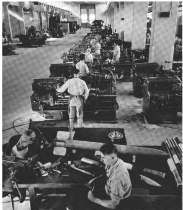
Michelson Laboratory machine shop, May 1948. Laid out on the front table are components of the 5.0-Inch High-Velocity Aircraft Rocket (HVAR).
