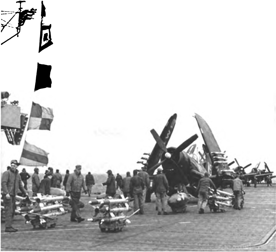
Navy and Marine Corps ordnancemen loading Holy Moses rockets and napalm on F4U-4B Corsair fighter-bombers on the deck of Badoeng Strait (CVE-116) during operations off Korea, December 1950.
