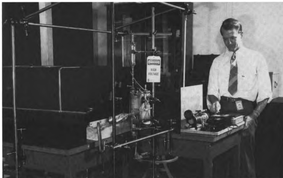
Spectrograph to measure features of the airglow spectrum.
