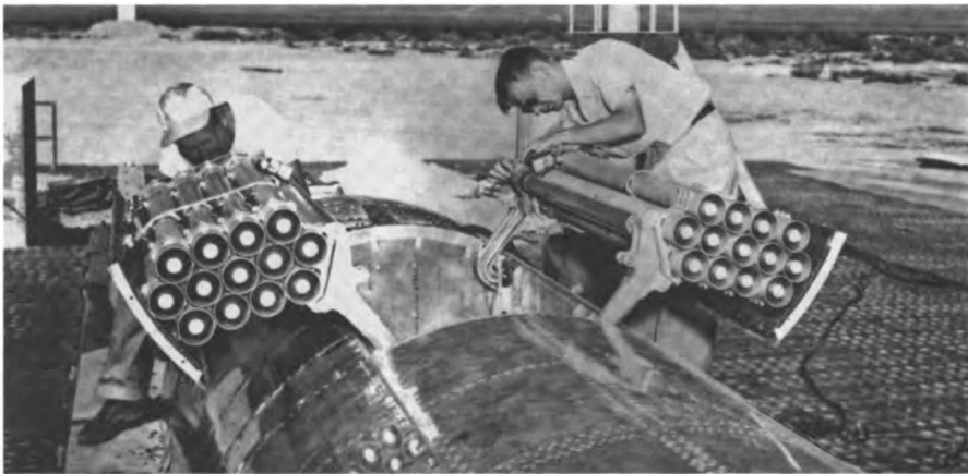
Sled preparations for rocket-launcher test on B-4 Track.
