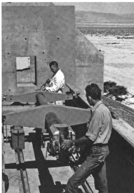
Loading a 3-inch gun to fire down the length of the new aeroballistics laboratory, 1 June 1953.
