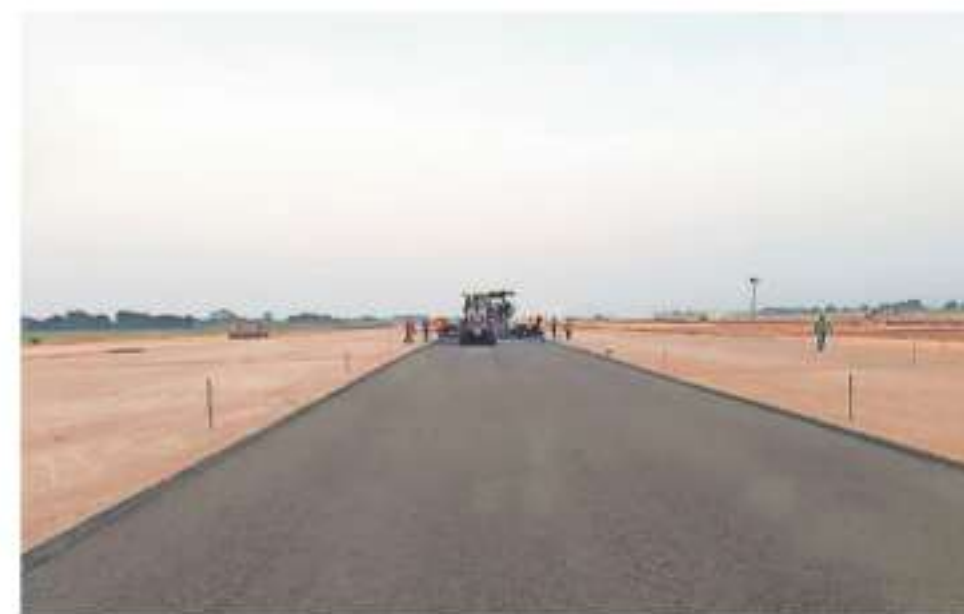
Work on the runway is almost 70% complete, said officials
