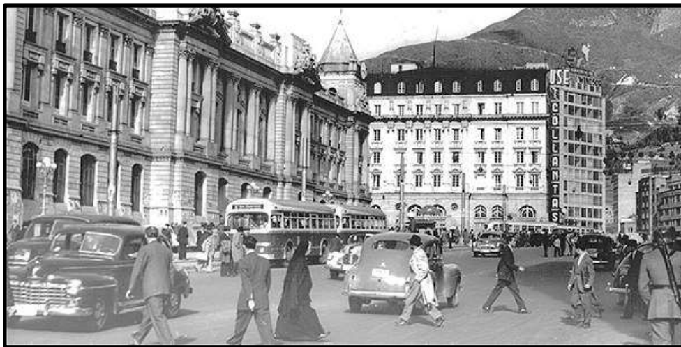
An example of the buildings to be demolished, Jiménez de Quesada Avenue, 1950
