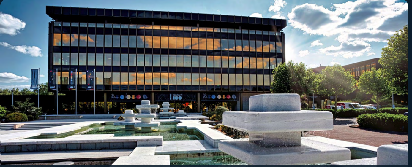
WATER AS PART OF THE ARCHITECTURE.
