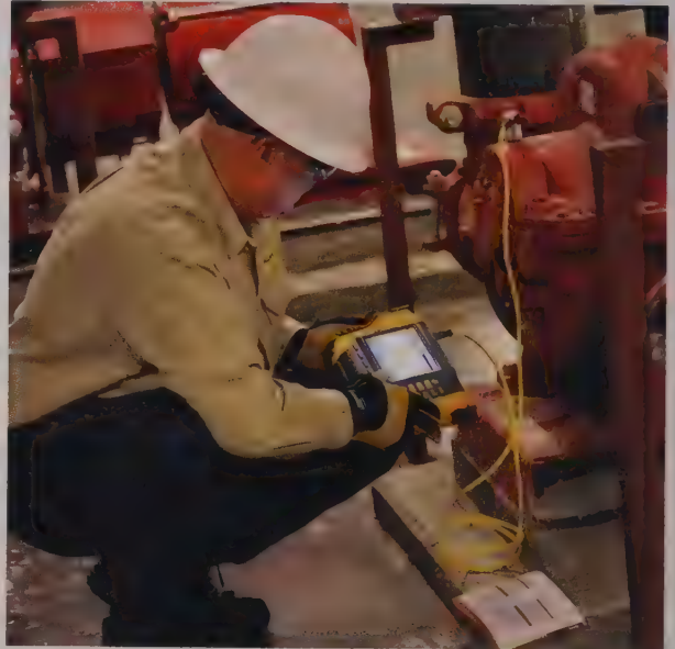
Vibration analysis is a type of periodic maintenance used to analyze the condition of equipment.
