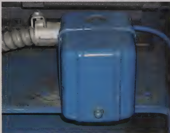
An air compressor uses a pressure switch to turn the compressor motor on or off based on the amount of pressure.
