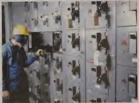
Figure 28-12. A motor control center provides a central location for the wiring, control, and troubleshooting of motor control circuits.
