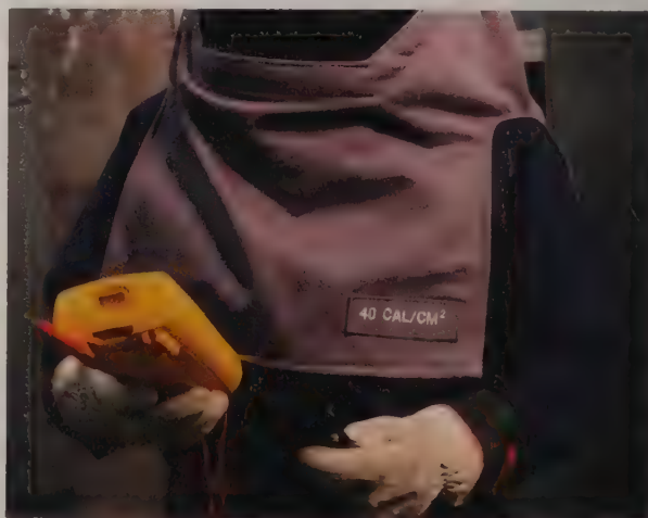
A digital multimeter (DMM) set to measure voltage is used to test circuit breakers.
