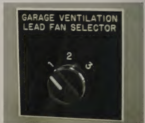
A three-position selector switch is a type of operator device that allows the user to select one of three circuit conditions.
