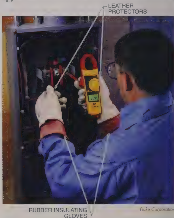
Figure 4-12. Hand protection includes gloves worn to prevent injuries to hands caused by cuts or electrical shock.
