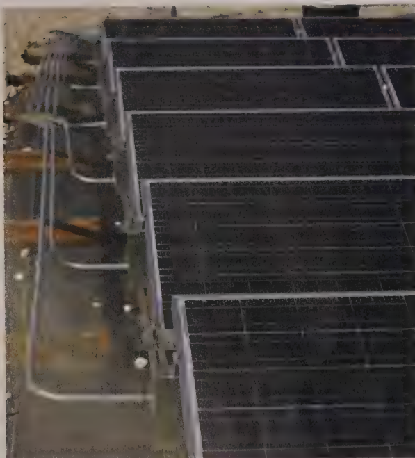
A photovoltaic cell is a semiconductor device that converts light energy directly to electrical energy.
