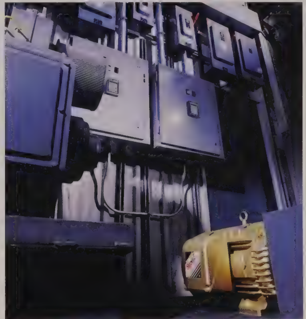
Figure 19-5. Primary resistor starting uses a resistor connected in each motor line and a timer to short the resistors after the motor accelerates to a specified point.
