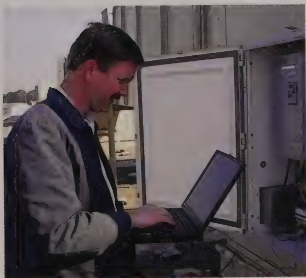
A PC can be used to program a programmable controller using application software.
