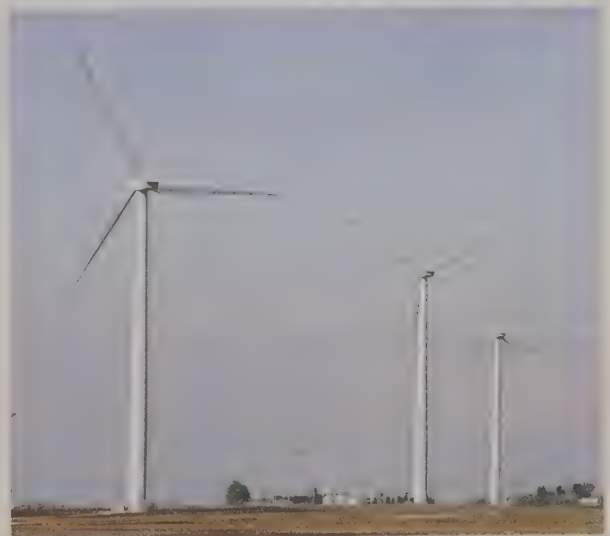
Distributed power generation systems such as wind turbines can be used as stand-alone systems or connect to a centralized power distribution system.
