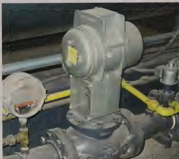
Flow switches are commonly used with boilers to detect if a fluid is moving.
