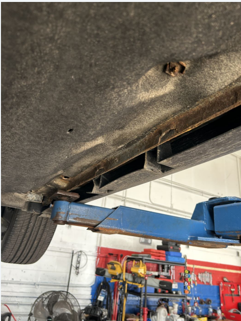
31 | Inspection photo Underbody covering and fasteners.
