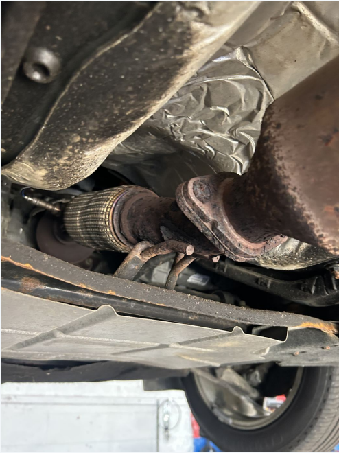
09 | Inspection photo Exhaust flex section and engine underside.
