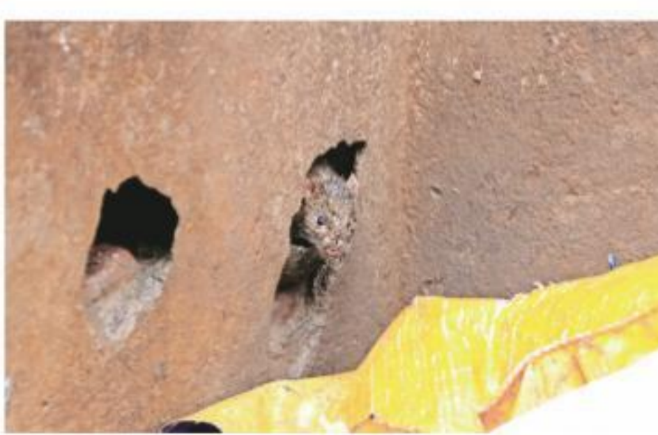
Rats have dug their way through several structures in the city, including at least two flyovers. Shashi Ghosh
