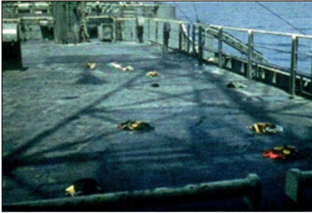
Forward deck house showing rocket holes plugged with rags
