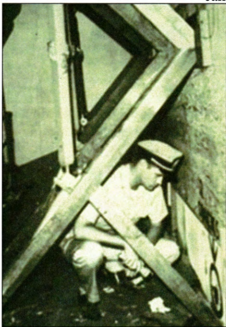
Damage Control Officer Ensign John Scott examines shoring
