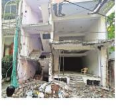
The building was demolished Thursday
