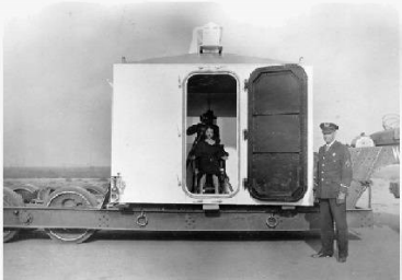
Gas chamber door, Colorado
