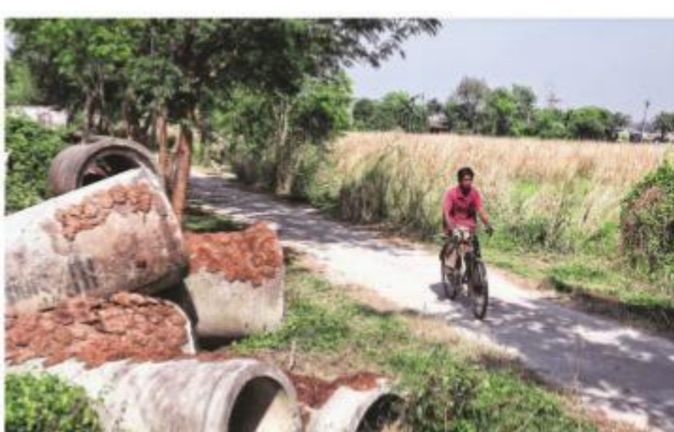
Abandoned pipes at the site in Singur. Partha Paul
