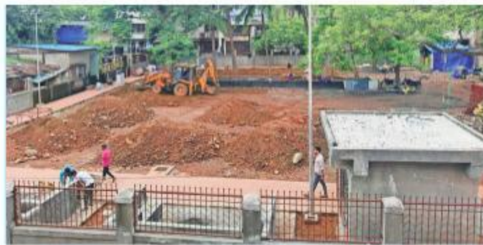
The under-construction Gandhi Maidan in Mumbai. Express
