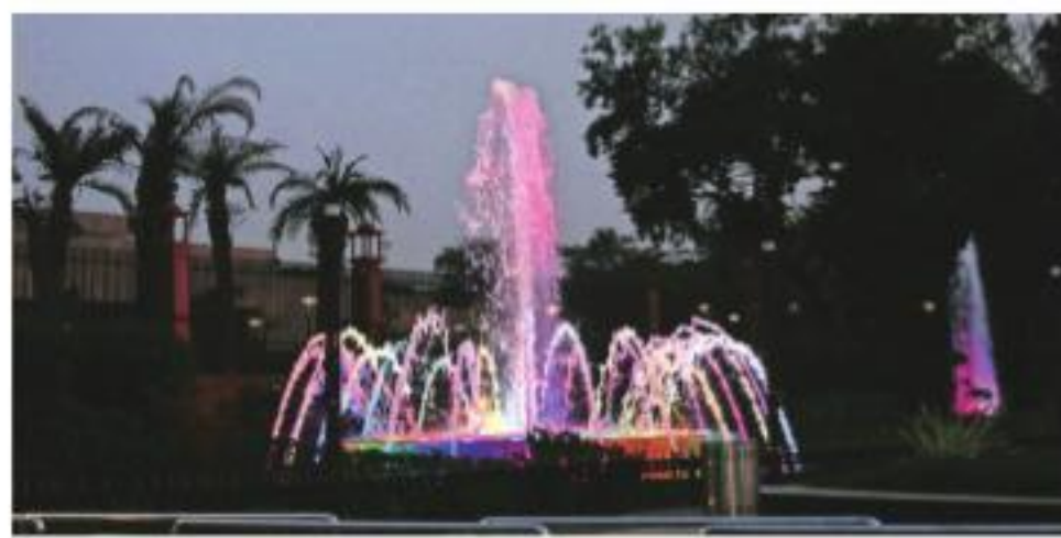
After the G20 Summit, nozzles installed inside the fountains, wires and ornamental lights were stolen by thieves. File
