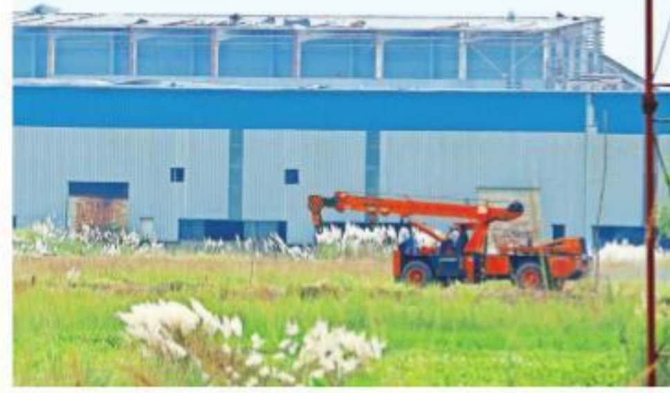
Dismantling work at the Singur Nano plant in 2016. Express File
